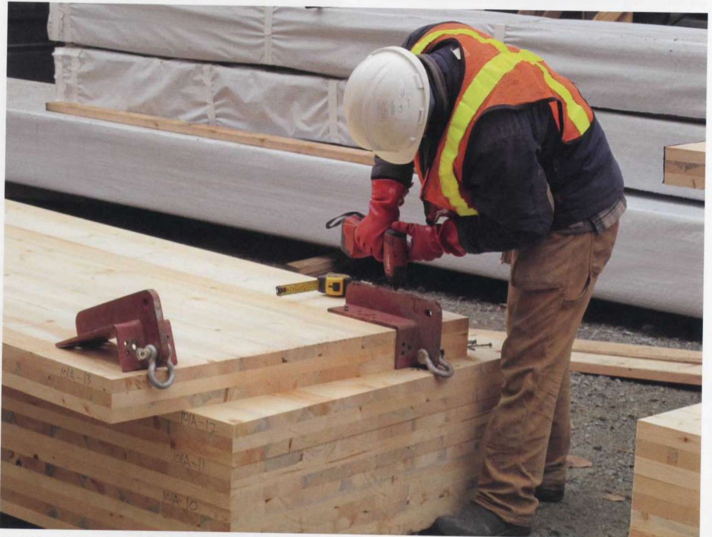
3.1.9 CLT panels being prepared for lifting. See BioEnergy Research and Demonstration Project for more information. Source: McFarland Marceau Architects
