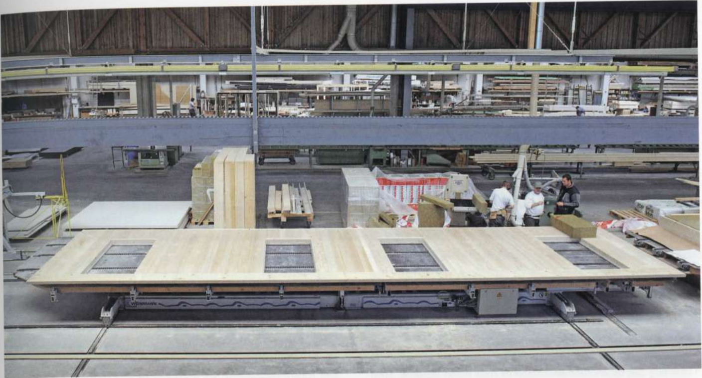
3.1.19 Solid wood wall prior to factory installation of gypsum board, insulation and exterior cladding. See H8 case study for more information. Source: Huber & Sohn
