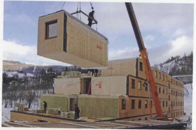
3.1.8 Modular CLT housing for 2005 Olympic Games in Torino. Source: KLH
