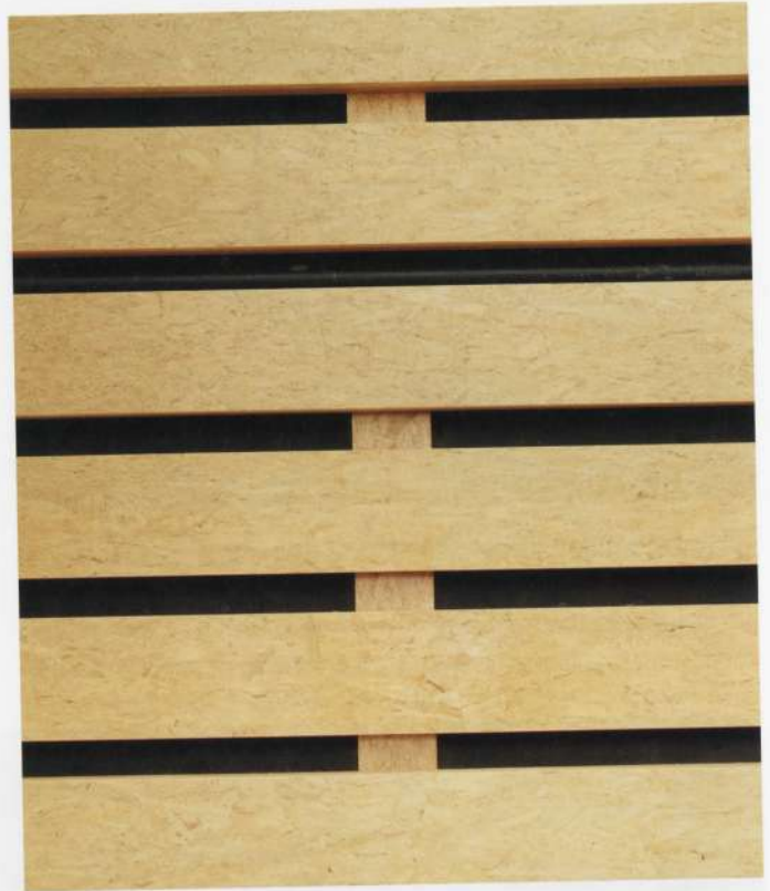
3.1.6 Laminated Strand Lumber used for ceiling at North Vancouver City Hall. See case study for more information. Source: Michael Green Architects
